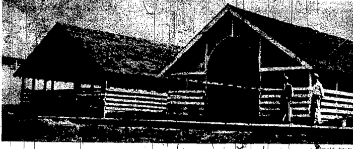
Fair board members are shown above inspecting new improvements at the Wayne County fairgrounds. Rollie W. Ley, director and H. B. Craven, president of the board, are at the right, and checking the hog loading and judging platform. The 85x20 cement slab is just part of the new improvements being made for the four-day event starting Sept. 12.
